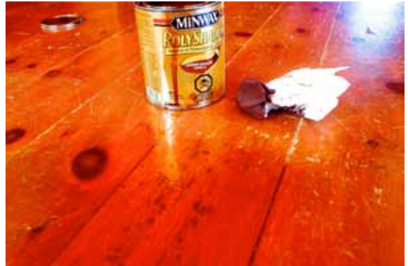
The area in the foreground has been stained during the restoration process. Areas behind have only been hand sanded, still awaiting stain.
