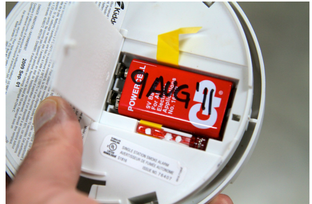
The installation date written on this smoke alarm battery takes the guesswork out of timely replacement. Photo credit: Steve Maxwell
